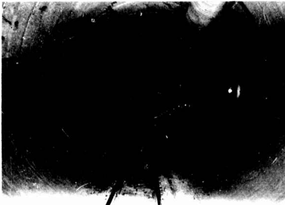
FIG. 16. Unlined Tunnel Driven in One Pass Through Sandstone. The tunnel is 19 to 21 feet in diameter depending on local rock conditions (Farmington).
